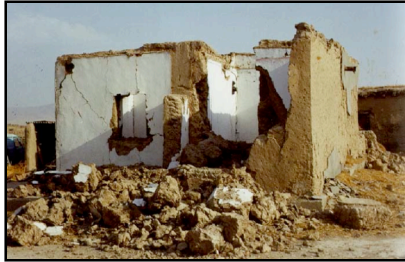
Damage to an adobe building in the January 2000 Kamashi Earthquake, Uzbekistan, (Khakimov Sh.A., Nurtaev B.S.)
